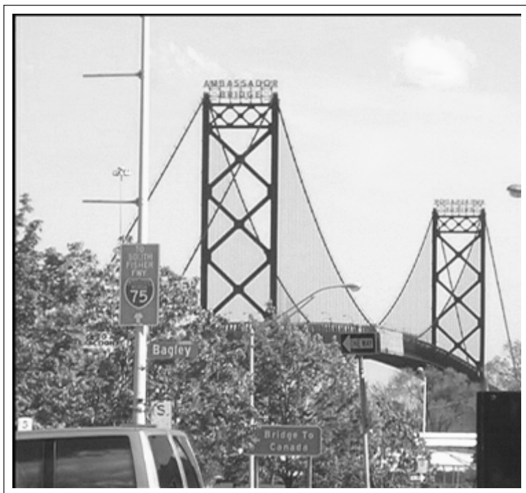
STILL PHOTO 1: DETROIT BRIDGE
